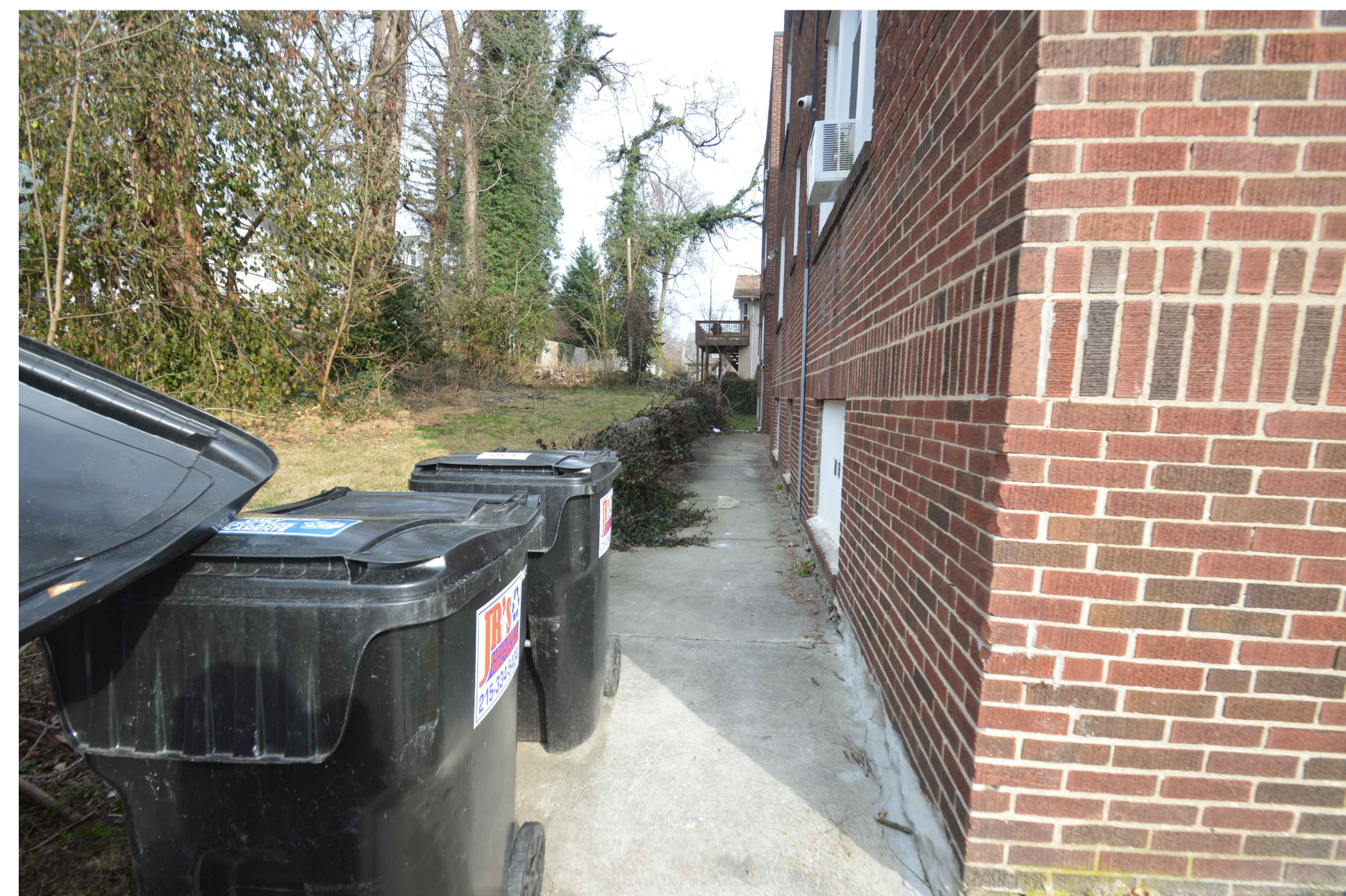
Rear Western Facade
