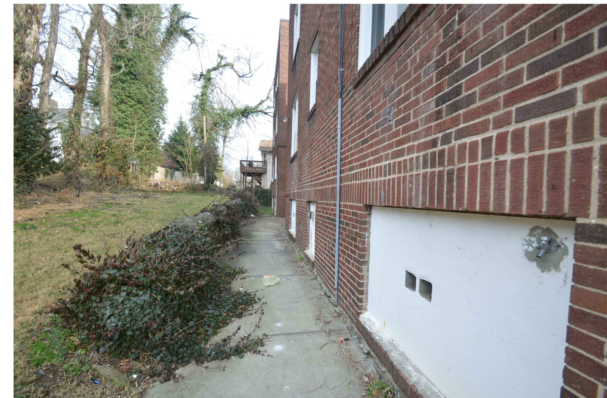
Rear Walkway to Courtyard
