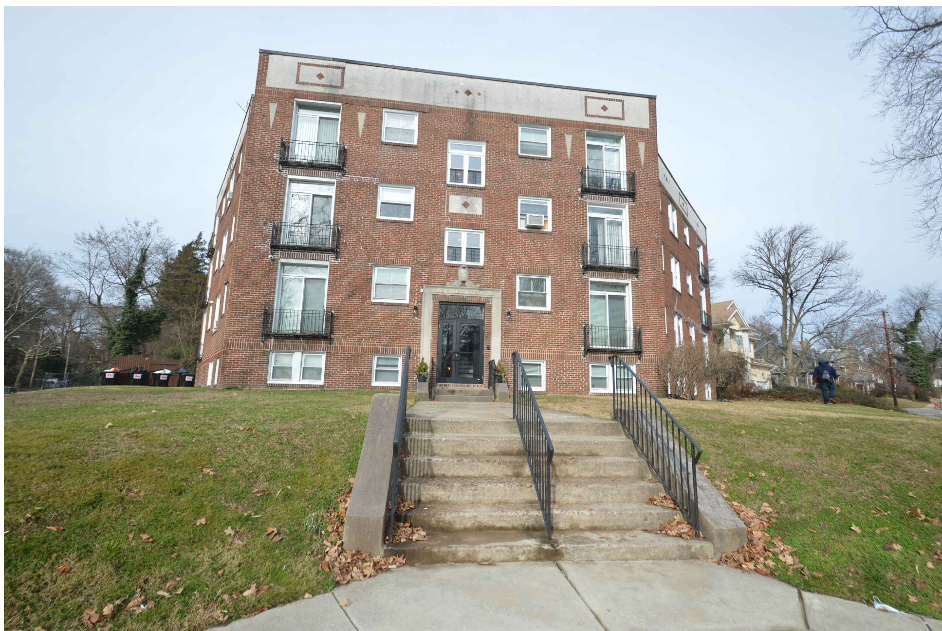
Approach to Building
